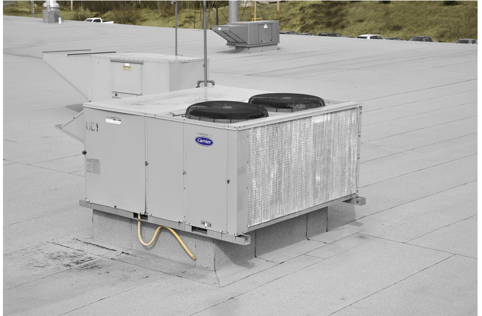
Figure 4. Typical air-handling unit.
