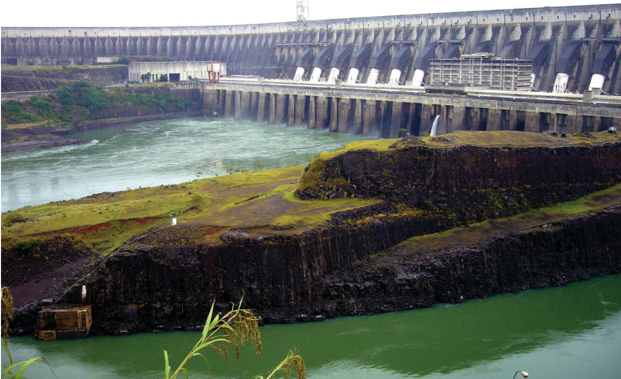
Figure 27. The Itaipu Dam is located on the Paraná River, at the border between Brazil and Paraguay. With an installed capacity of 14 000 MW, it is one of the world's largest capacity hydropower plants.
