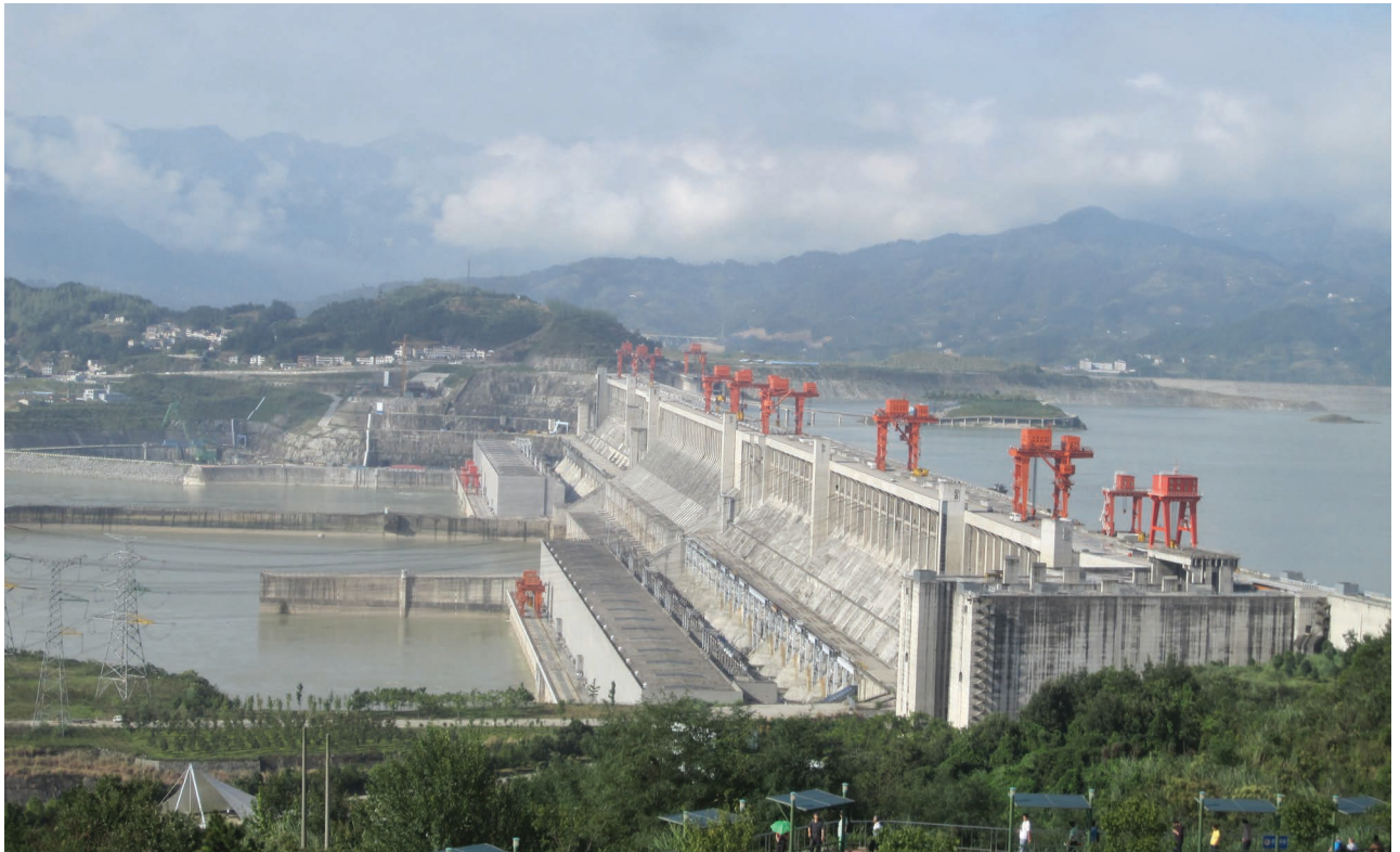
Figure 1. The Three-Gorges Dam on the Yangtze River in China has a total installed capacity of 20 300 MW (photo courtesy of Le Grand Portage).
