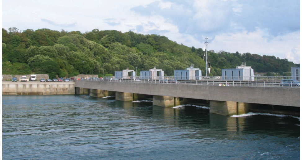
Figure 6. Tidal hydropower plant in Rance, France. It is the world's first large-scale tidal hydropower plant and has a peak power rating of 240 MW (photo courtesy of User:Dany 7C3).
