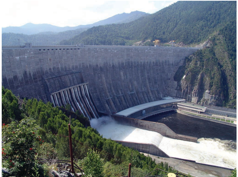
Figure 3. The Sayano-Shushenskaya dam hydropower plant in Russia is one of the largest in the world. Its installed capacity is 6400 MW (photo courtesy of MVValt).
