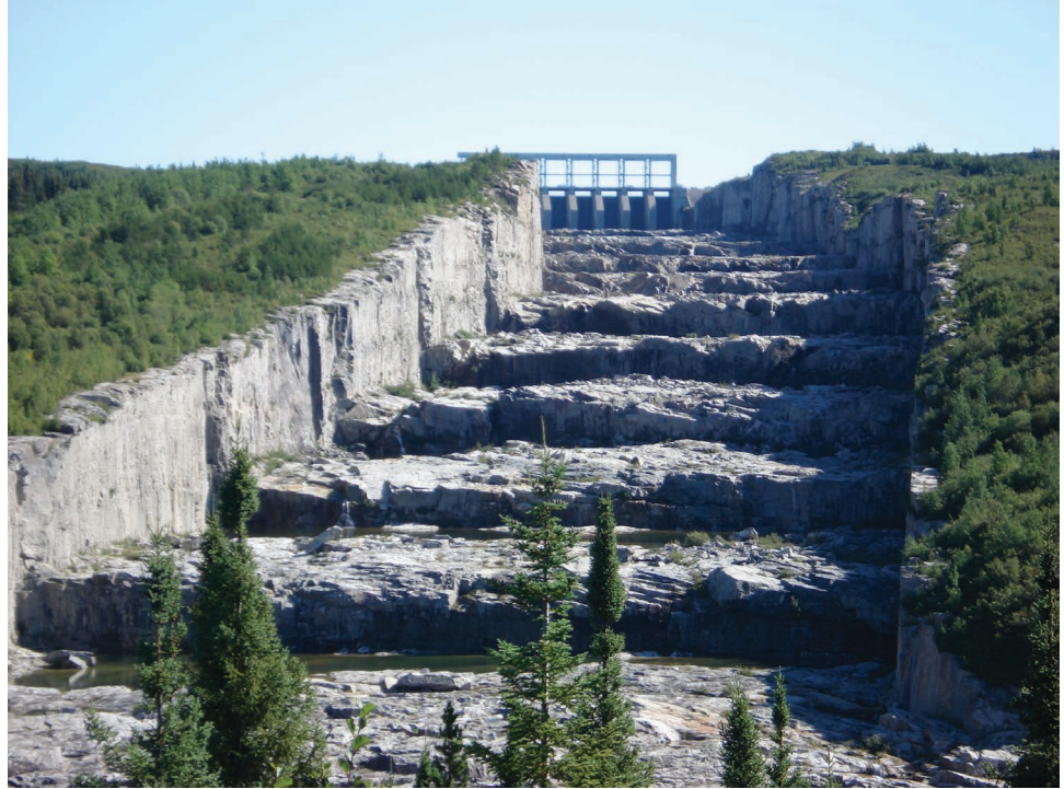
Figure 8. Water spillway from the Robert-Bourassa dam hydropower plant in the province of Quebec, Canada. With a total installed capacity of 5600 MW, the Robert-Bourassa dam hydropower plant is among the largest in North America (photo courtesy of fargomeD).
