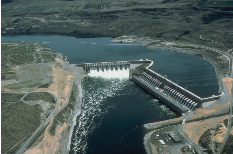
Figure 5. View of the Chief Joseph Dam hydropower plant on the Columbia River in the state of Washington, USA. The Chief Joseph Dam is a run-of-river hydropower plant with a capacity of 2600 MW.
