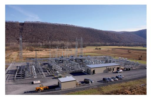
Figure 37. SVC substation in Maryland, USA. This substation was installed primarily to enhance the reliability of the heavily loaded power transmission lines in the area (photo courtesy of ABB).
