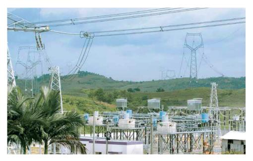
Figure 30. SVC substation in Pingguo, China (© Siemens AG 2012, all rights reserved).
