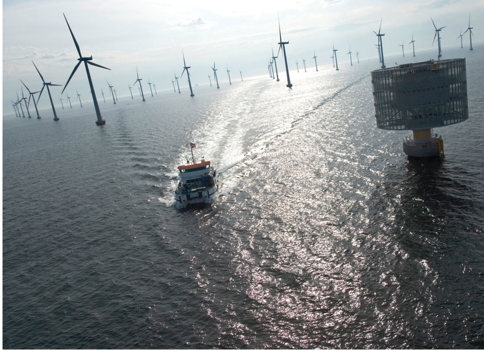
Figure 2. Voltage-source converter (VSC) devices such as STATCOMs are used in offshore wind farms to ensure that the quality of the power produced by the wind farm is optimal. The above picture shows the Lillgrund wind farm in Sweden (© Siemens AG 2012, all rights reserved).
