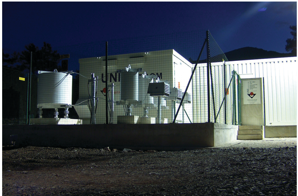
Figure 20. The voltage across a STATCOM designed for automatic voltage compensation is controlled using a voltage control loop. This ensures that the voltage across the STATCOM is maintained virtually constant (© Copyright 2012 Guc Kalitesi).
