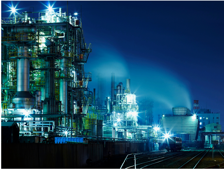
Figure 2: Industrial applications often include large electric loads that require a substantial amount of reactive power to operate, thereby resulting in a low power factor. To comply with the power factor limit imposed by the electricity provider, some means of correcting the power factor (e.g., an APFC system) at the electric power entrance is required in most industrial applications.
