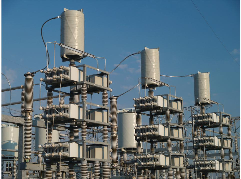
**Figure 11.** Banks of capacitors are often used in power transmission substations. Capacitors such as these have a very high capacitance value.
