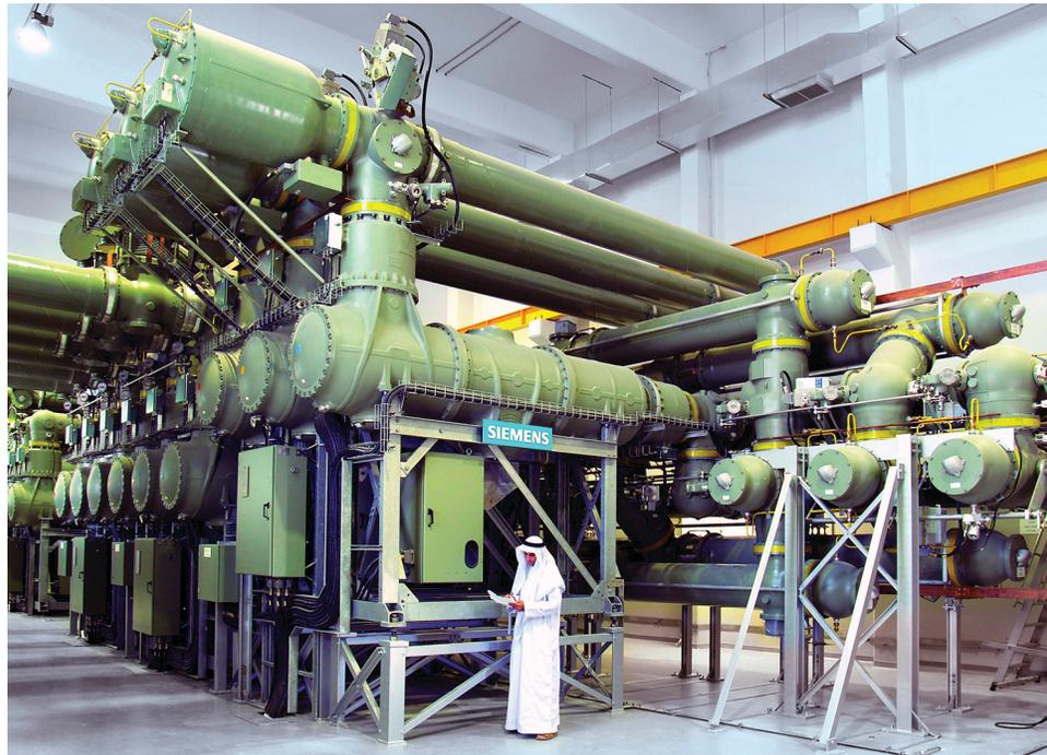
Figure 34. Gas-insulated 400 kV high-voltage switchgear at a substation in Abu Dhabi, in the United Arab Emirates. This substation contains 24 switchgear bays at 400 kV and 28 at 132 kV, making it one of the largest in the world (© Siemens AG 2014, all rights reserved).
