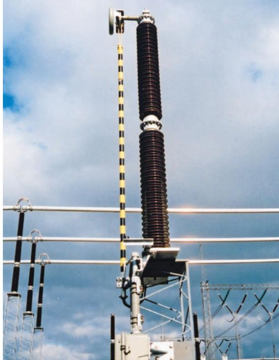
Figure 31. A grounding switch in the closed state. The black and yellow arm of the switch is bonded to ground (© Siemens AG 2014, all rights reserved).
