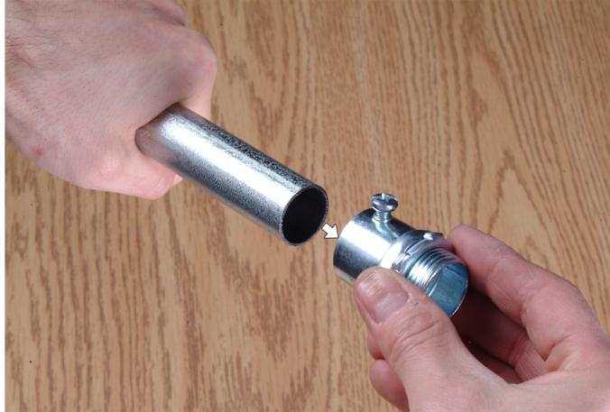
**Figure 34.** Installing a fitting to one end of a piece of EMT.
