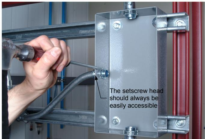
**Figure 35.** Securing an EMT and fitting assembly to an enclosure or box wall using a lock nut.
