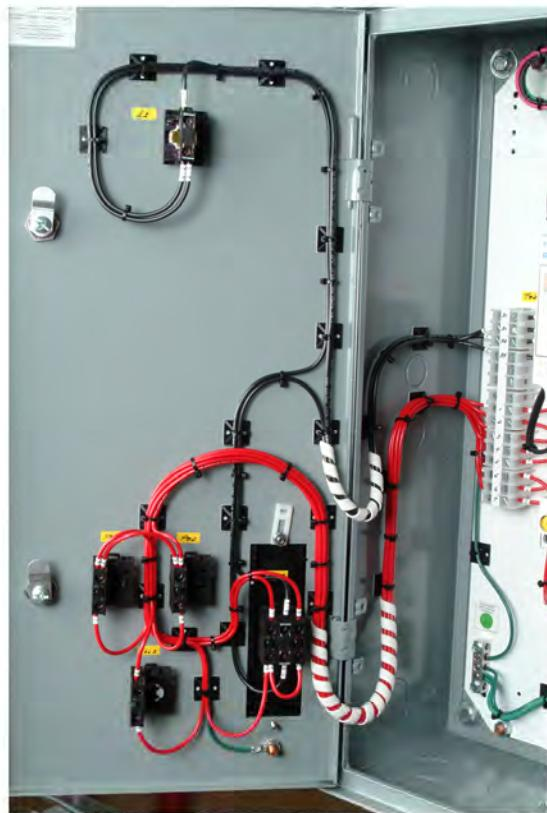
Figure 2-4. Connections of the AC motor drive controls and pilot lights.
