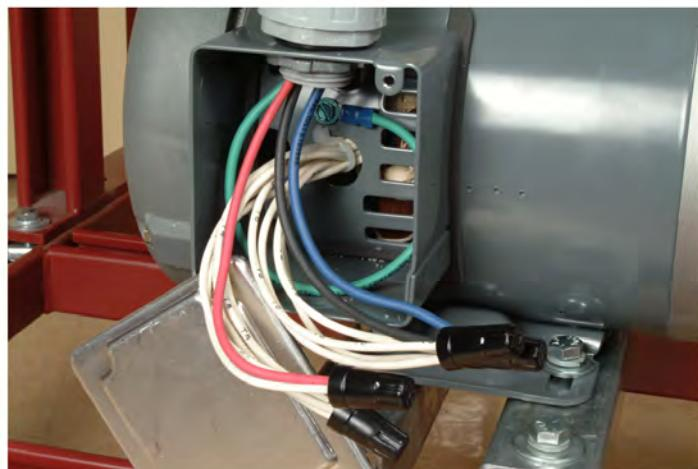
Figure 2-6. Connections at the 1/2-HP, three-phase induction motor.
