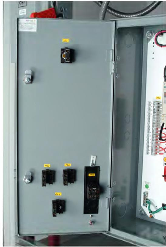
**Figure 2-3. AC motor drive controls and pilot lights installed on the new MCE door panel.**
