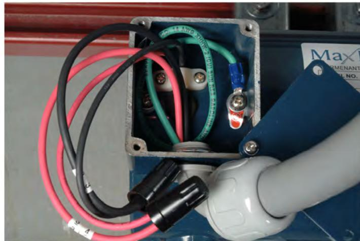
Figure 1-8. Connections at the 1/2-HP, permanent magnet DC motor.
