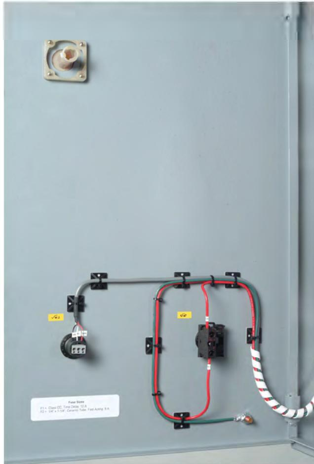
**Figure 1-6. Connections of the DC motor drive controls.**
