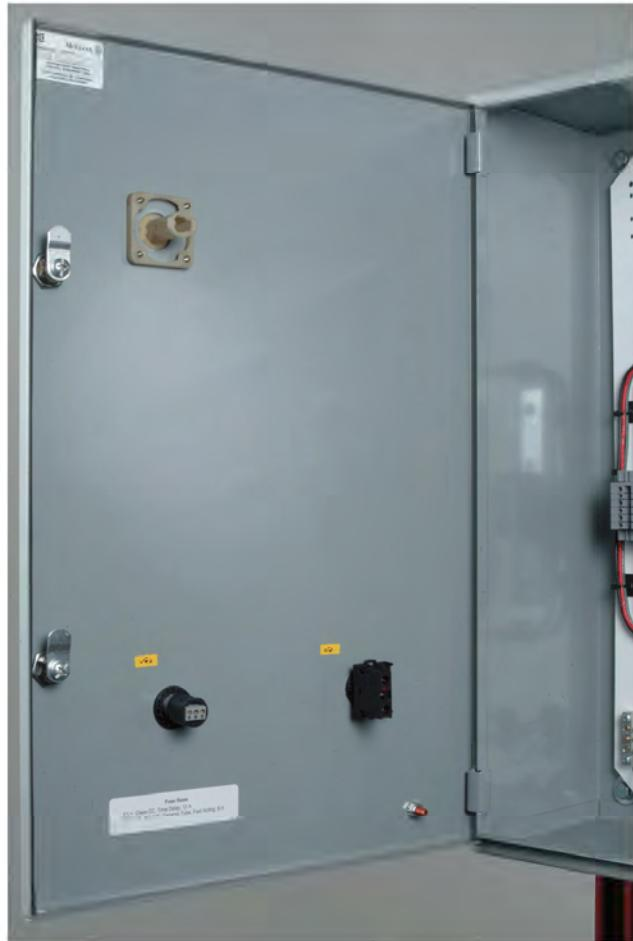
Figure 1-5. DC motor drive controls installed on the MCE door panel.
