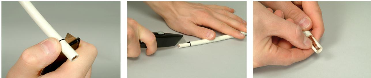
Figure 16. Strip the end of the service-entrance conductors.
