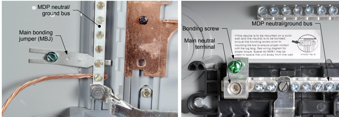
**Figure C. MDP enclosures equipped with either a bonding screw or a main bonding jumper (MBJ).**
