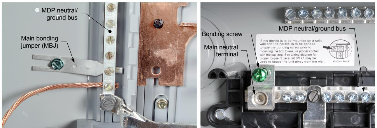
Figure 19. MDP enclosures connected to the neutral/ground bus using either a MBJ or a bonding screw.
