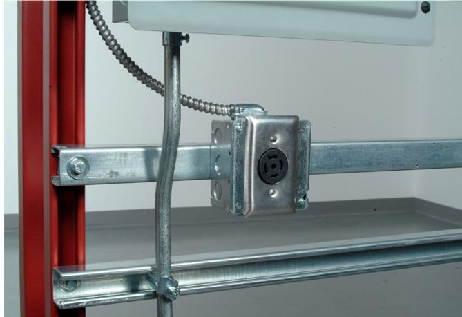
Figure 28. Three-phase receptacle with faceplate installed.
