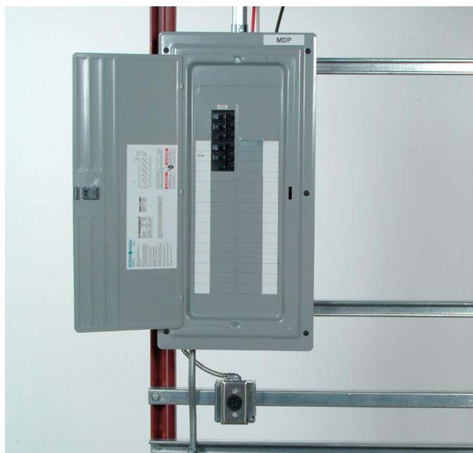
Figure G. MDP with the front panel installed and labels applied.
