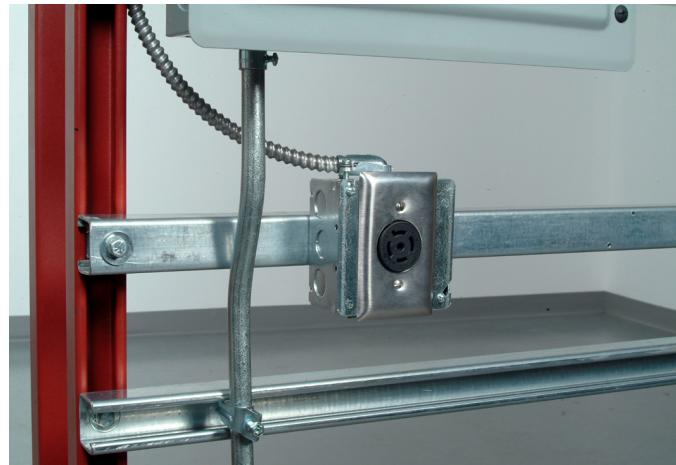
Figure H. Three-phase receptacle with faceplate installed.
