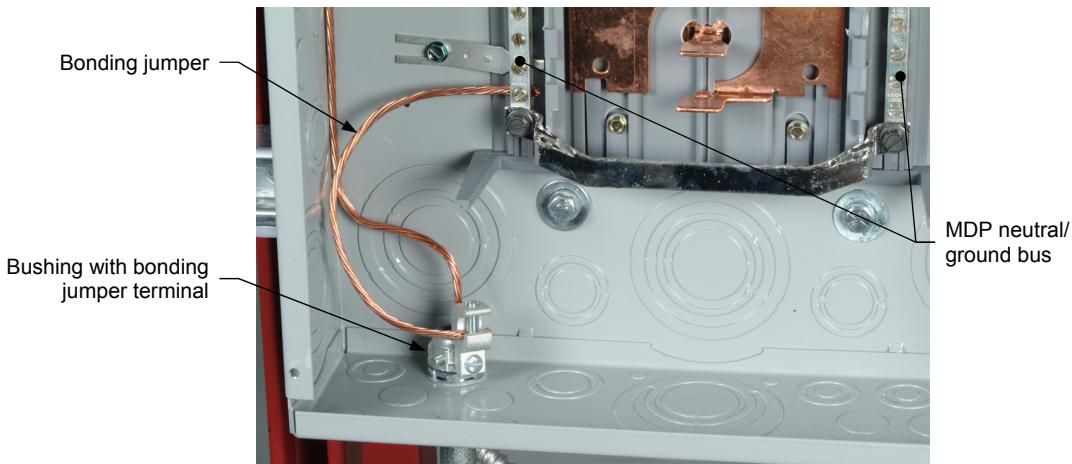
Figure 20. Bushing with a bonding jumper terminal connected to the MDP neutral/ground bus.
