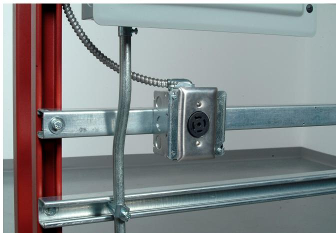
Figure 28. Three-phase receptacle with faceplate installed.
