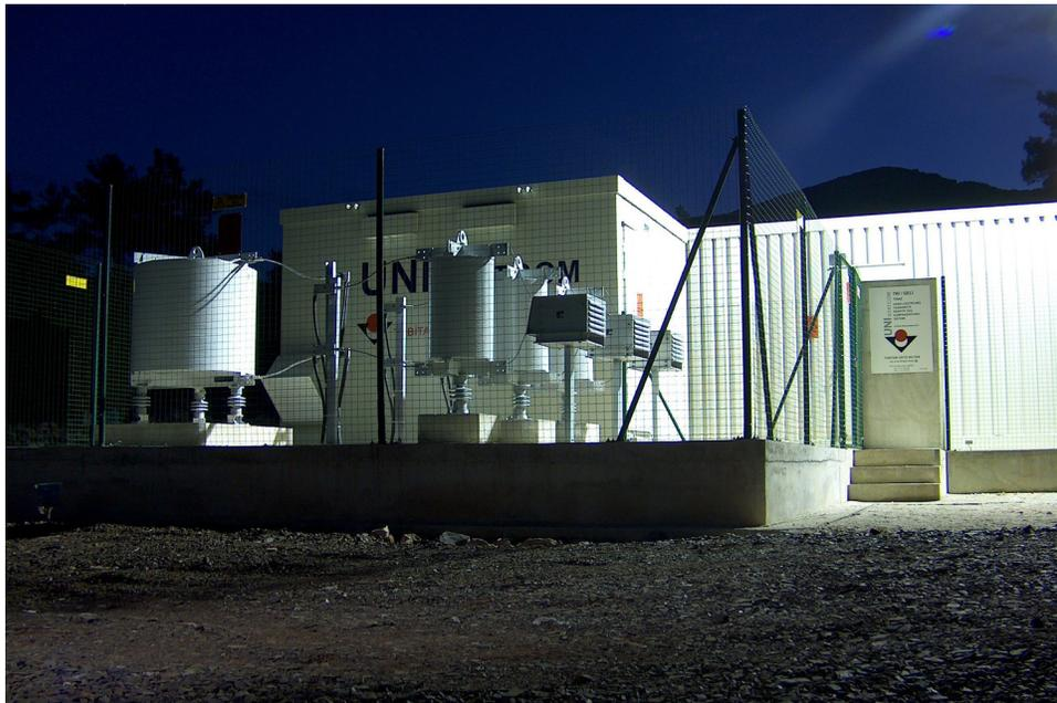
Figure 10. STATCOM substation in Turkey (© Copyright 2012 Guc Kalitesi).
