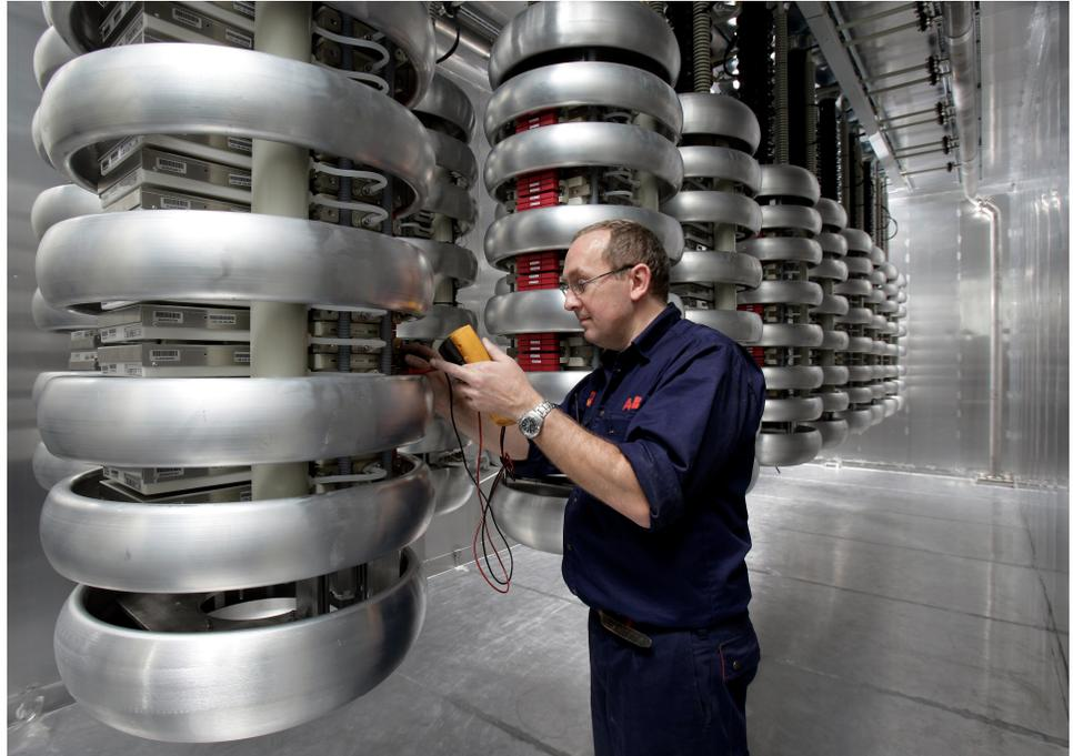
**Figure 11. VSC HVDC converter valves in an offshore wind farm power generating station north of Germany (photo courtesy of ABB).**
