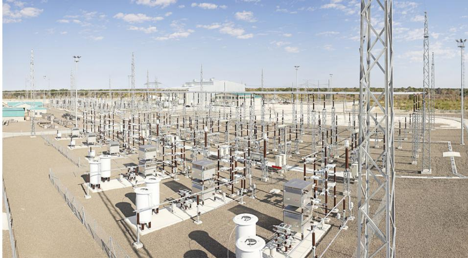
**Figure 12.** 350 kV VSC HVDC substation linking the ac power network of northeastern Namibia to that of central Namibia. This substation also helps in stabilizing both networks (photo courtesy of ABB).
