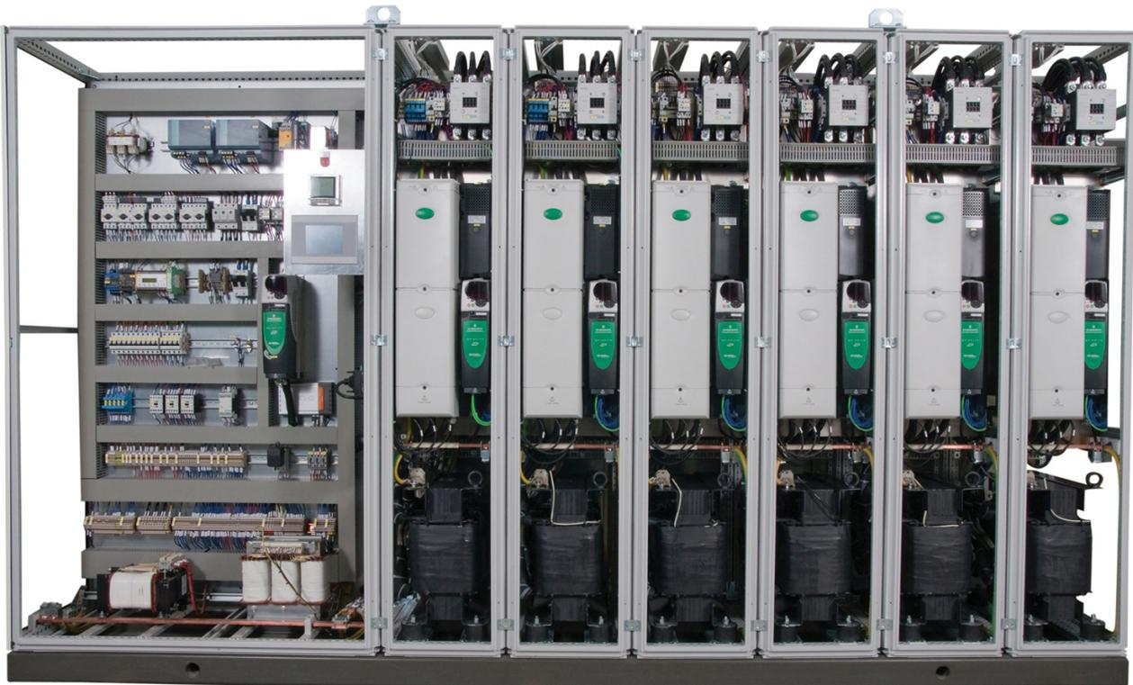
**Figure 15.** Three-phase PWM rectifier/inverter used for dc-to-ac power conversion in a solar power plant.
