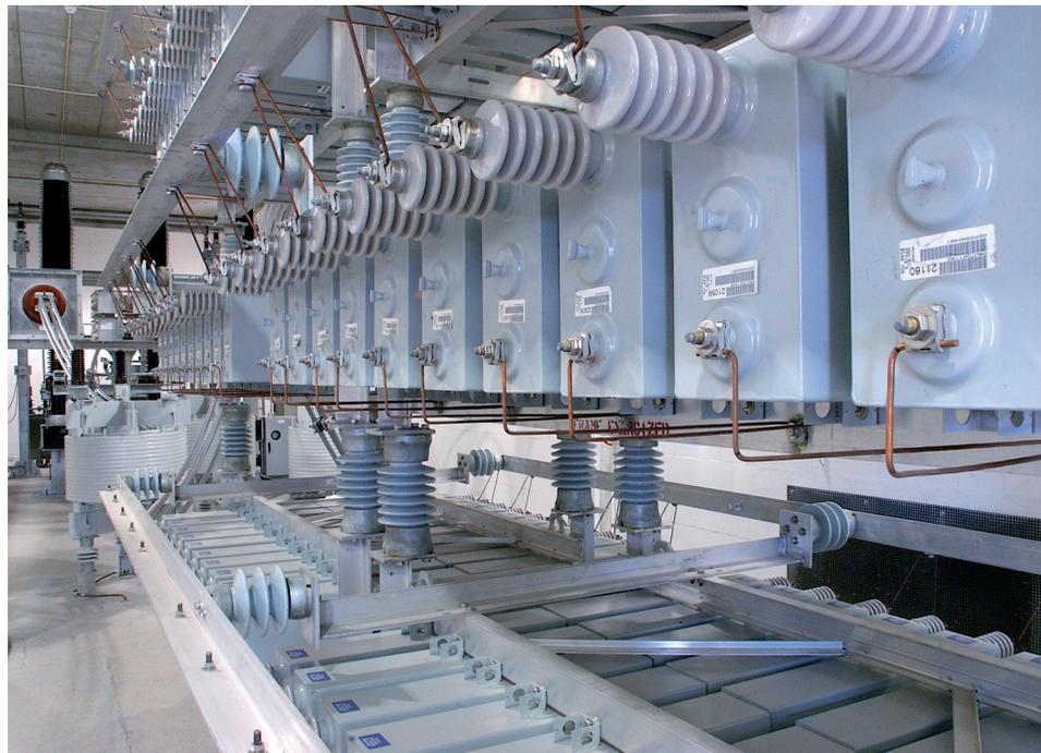
**Figure 1.** Indoor view of a static var compensator (SVC) substation in Denmark. (© Siemens AG 2012, all rights reserved).
