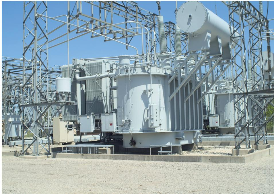
**Three-phase transformer bank used for power distribution.**
